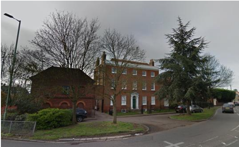
Fig 6: Google Maps image of properties 41 – 43 Upper Tilehouse Street (grade II). Available at: http://maps.google.co.uk [Accessed: 9 January 2024].
